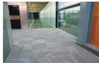
Floor covered with Carpet Tiles
