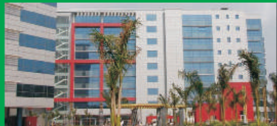
Olympia Technology Park, Chennai Insulation: Wall - AAC Blocks
