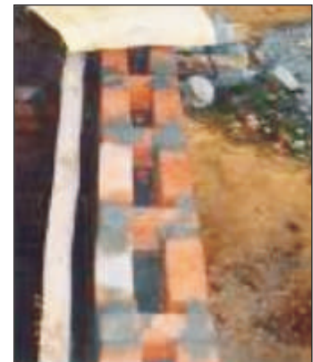
Rat trap bond filled with glass wool
