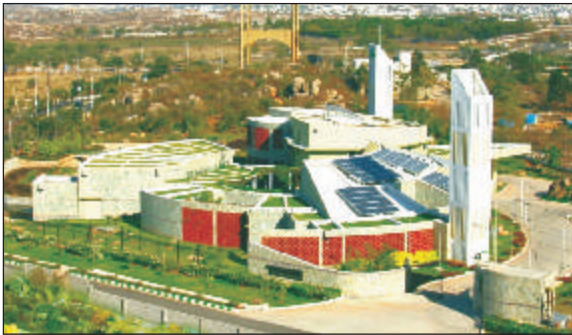
CII – Sohrabji Godrej Green Business Centre, Hyderabad Insulation: Wall - AAC Blocks, Roof: Extruded Polystyrene
