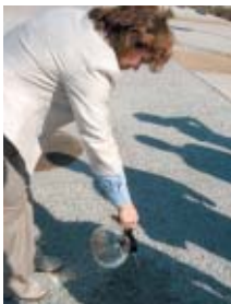
Concrete pervious car parking area
