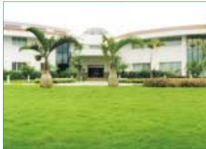
Vestas Wind Technology Chennai (LEED Gold)
