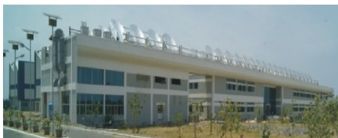
Turbo Energy Limited (TEL) R&D and Administration Block at Chennai
