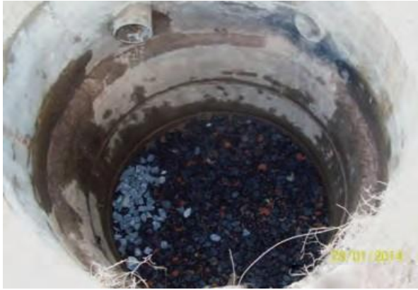
Rainwater recharge pit
