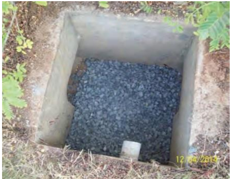
Rainwater collection chamber with filtration
