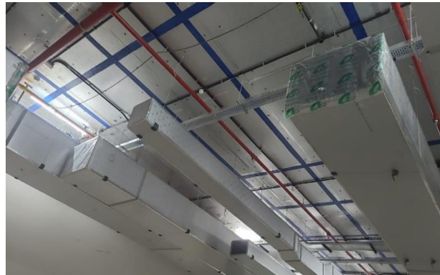
Protect ducts and equipment by sealing
