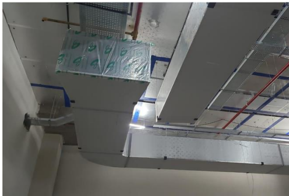
Protect ducts and equipment by sealing
