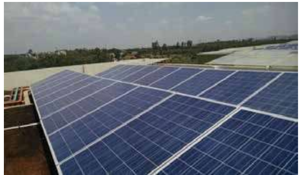
Centralized Solar-PV system for Street and Common area lighting
