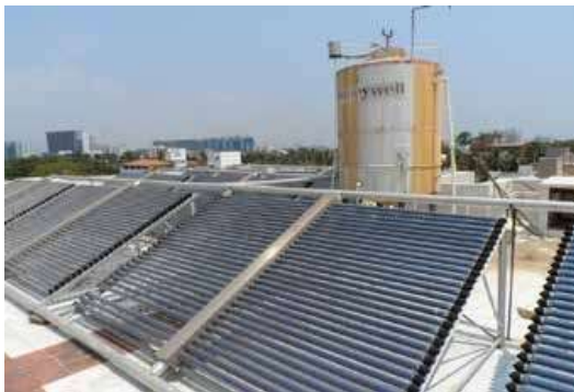
Centralized Solar Hot Water System
