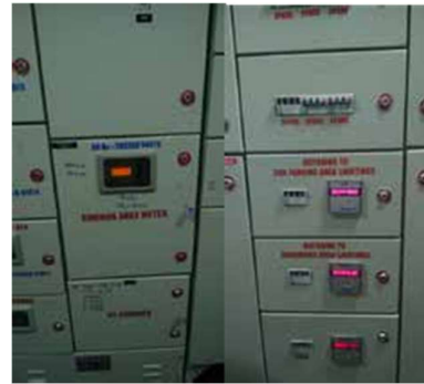
Energy Meters measuring Lighting and Equipment Loads
