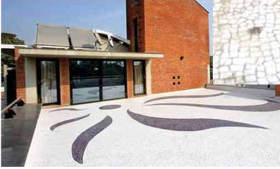
China mosaic tiles installed on Roof
