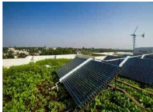
Individual Solar Hot Water System
