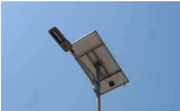
Stand Alone Solar-PV Street Lights
