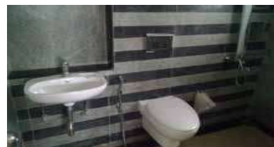
Water Closet with Dual Flush
