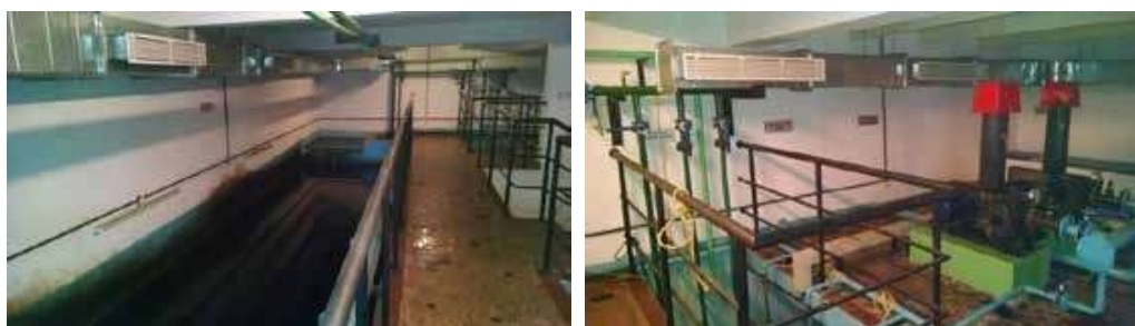
On-Site STP for treating waste water
