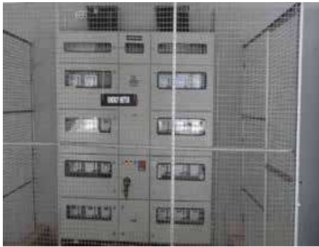
Energy Meters measuring Common Area Loads
